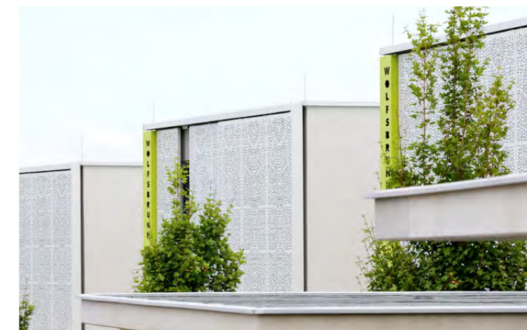
Terraced houses, Wolfsbrunn, perforated metal sheets
