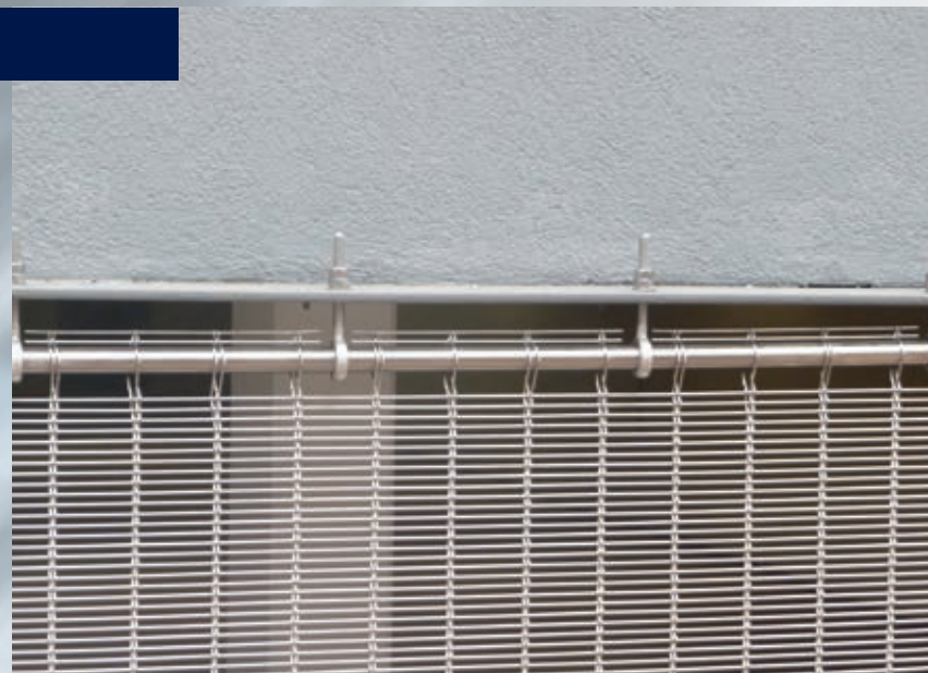
Top mounting: round bar with eyebolts.
