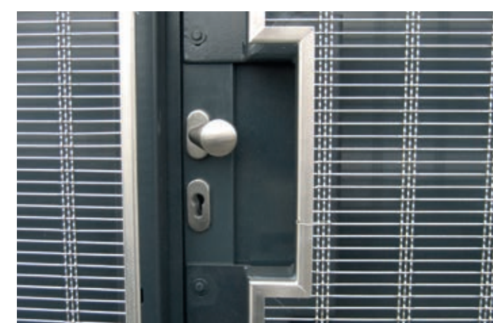
Mesh with edge protection profiles.
