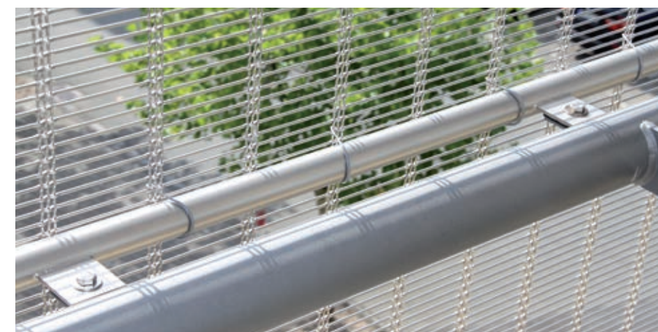
Intermediate mounting: round tube and wire connectors.
