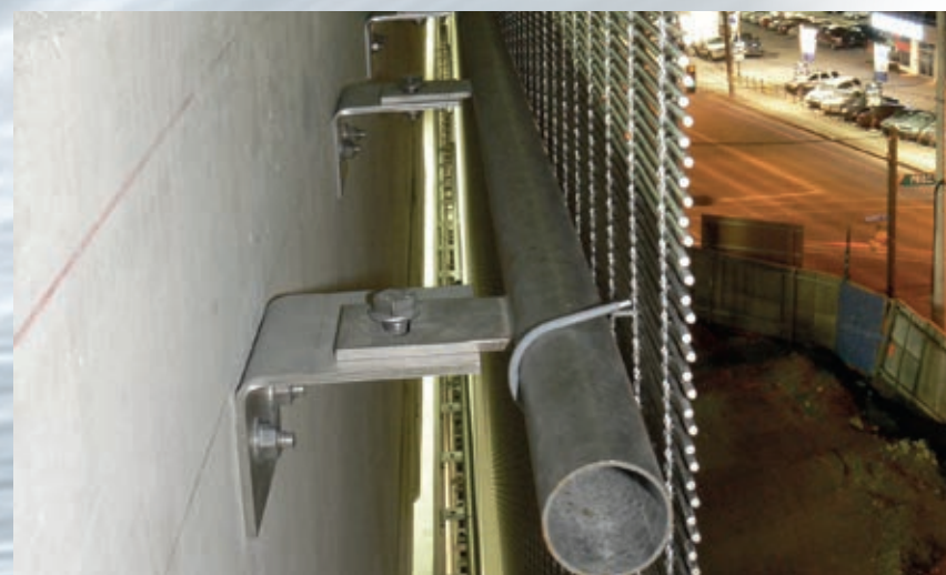
Intermediate mounting: round tube and wire connectors.
